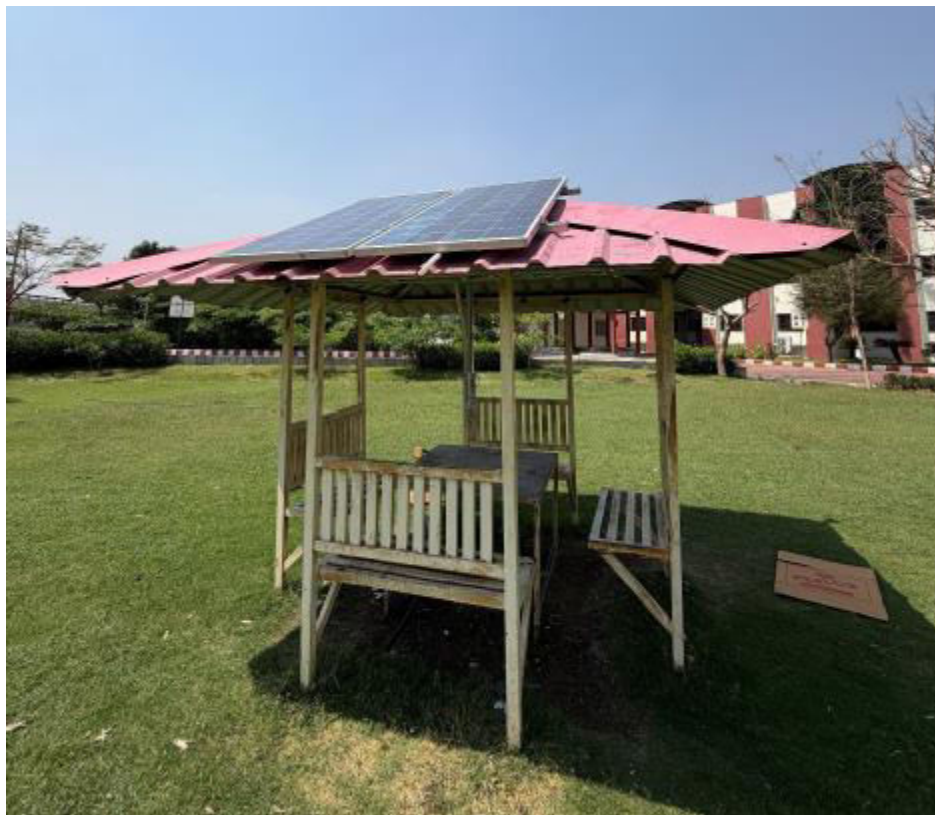
Figure 2.1 shows the installation phase of the Smart Solar Gazebo
